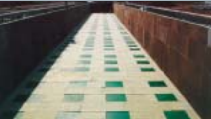
Figure 2: After installing the isolation (green)
