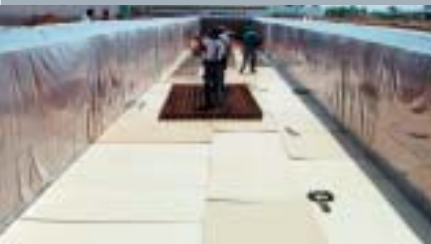
Figure 3: Block preparation for pouring the foundation
