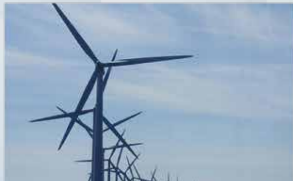
Lighting and Energy Poles
